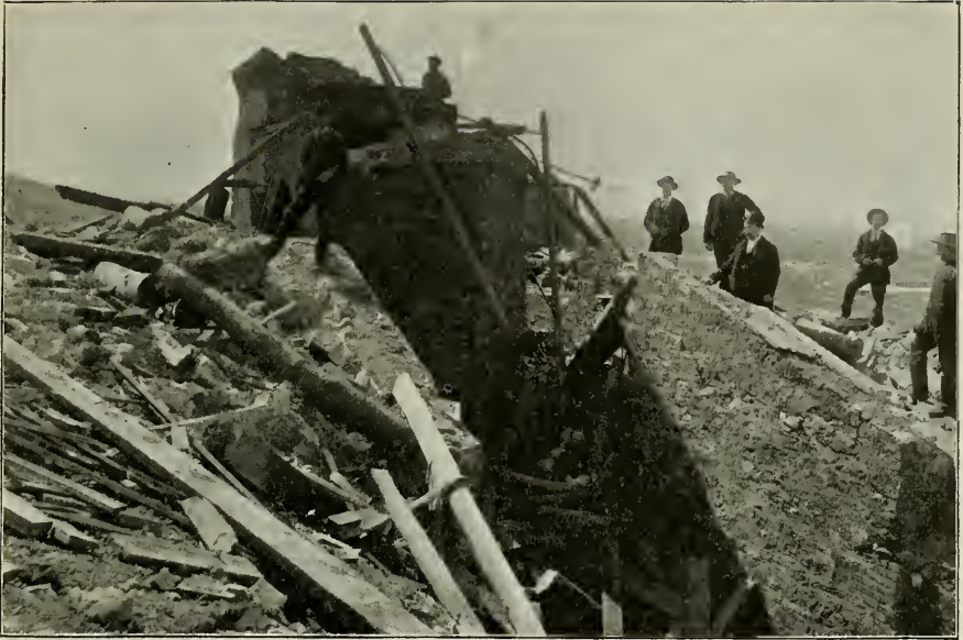
AIR FAN AND SHAFT NO. 5 MINE, ALMY, AFTER EXPLOSION.
